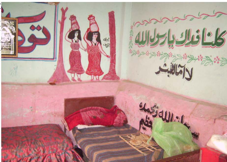
top: The view from the room of Shirihan Hamdi Mohamed Ahmed in Al-Shohba area of Al-Duwayqa, 9 February 2009. She told Amnesty International that the wooden ceiling of her room had collapsed after a rock fall.
