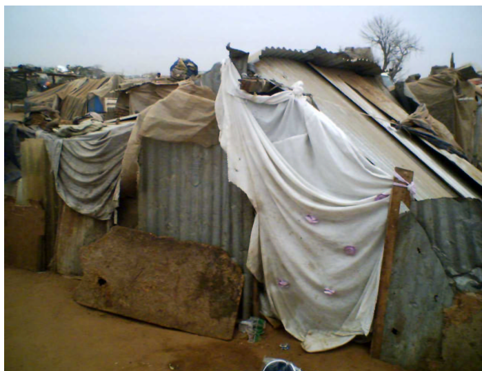
Shelter constructed from the ruins of demolished homes in Cambamba. Some residents were still living in such shelters at the time of writing. © Private, August 2006
