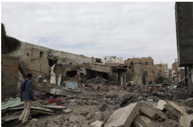
Destruction in the Mi'yad neighbourhood resulting from an airstrike on 13 June, killing five members of the al-Amiri family ©Amnesty International.
