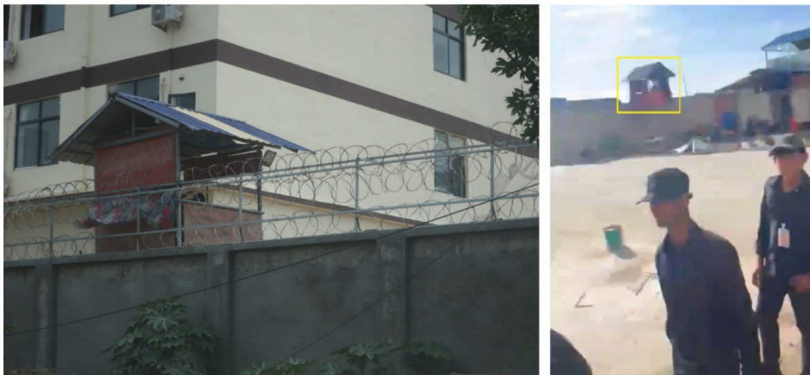
A picture taken by Amnesty International (left) and a frame of a video posted on social media by a security guard (right) show security guard towers with no capacity to look outwards at compound BA06. Source: Amnesty International, 2025
