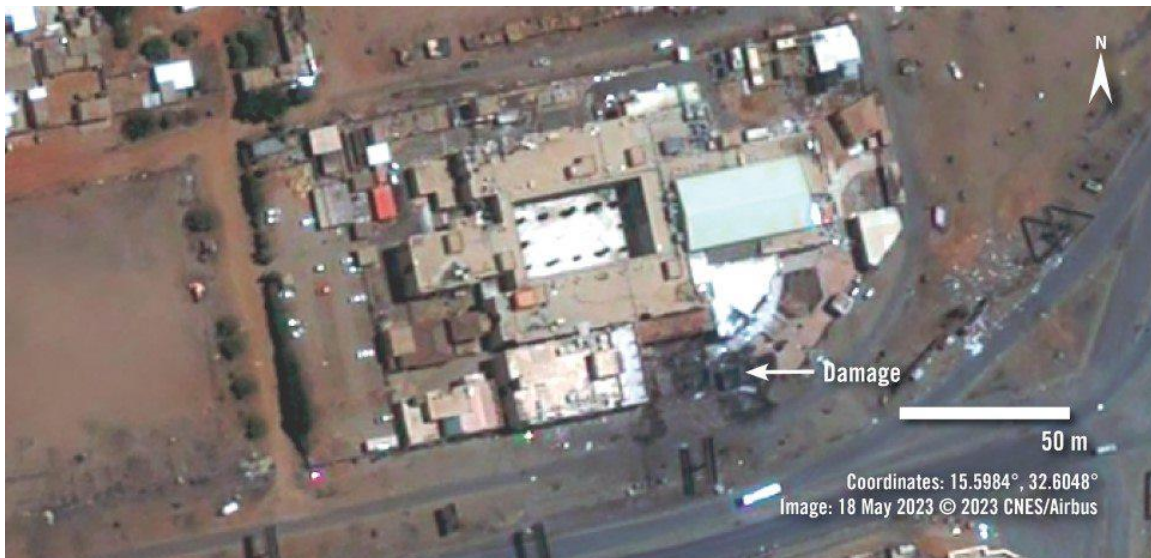
↑ On 18 May 2023, imagery shows the south side of the hospital has been heavily damaged.
