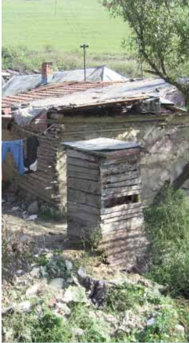
Outdoor latrine empties directly into river in Romani settlement.
