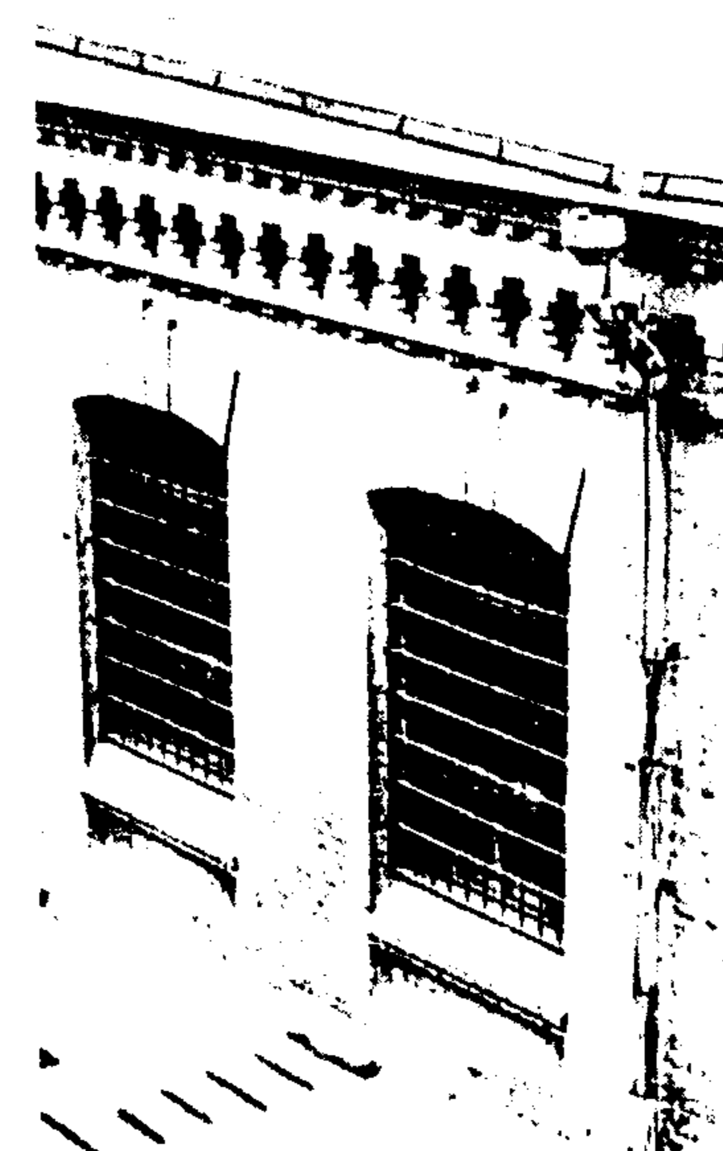
35 Some windows close up
