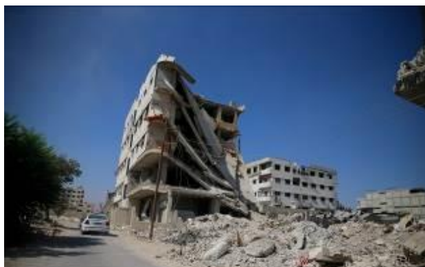
A building destroyed by bombardment by government forces in Zamalka [زملكا] in Eastern Ghouta in September 2013. © Mohammed Abdullah
