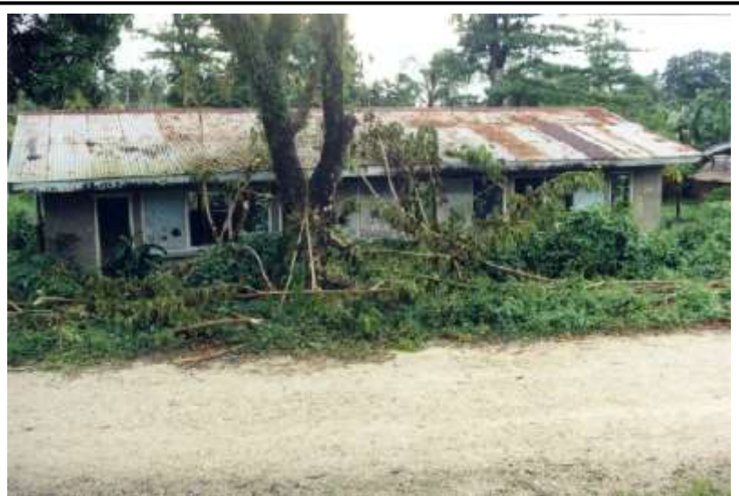
Malu'u Police Station staff housing, North Malaita, April 2004. © AI
