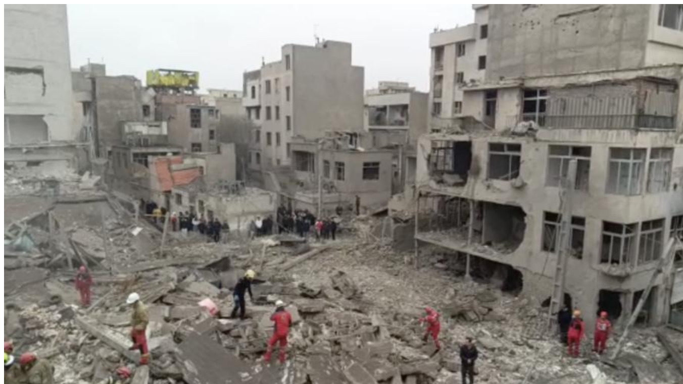
Still from a video that shows parts of the police station in Javadih destroyed, as well as destruction and damage to other surrounding buildings in Ghorbani street. © Sharghdaily
