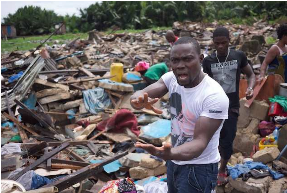
A former resident in Abonnema Wharf expressing anger at the demolitions on day 1, Wednesday 27 June 2012.
