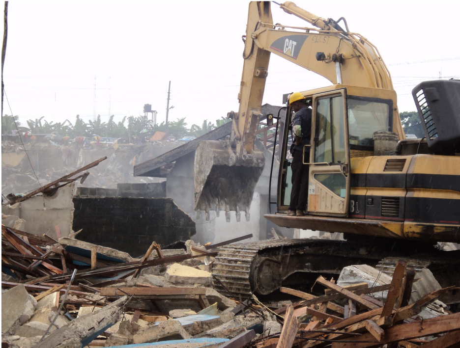
Excavator demolishing houses in Abonnema Wharf – Thursday 28 June 2012.
