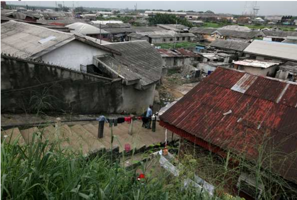
Abonnema Wharf before the demolition – 27 April 2011.
